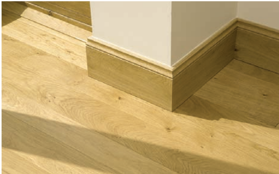
Oak flooring and skirting
