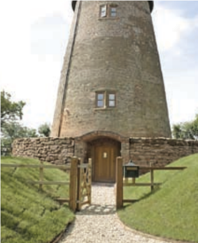
Windmill in Staffordshire, fencing and door
