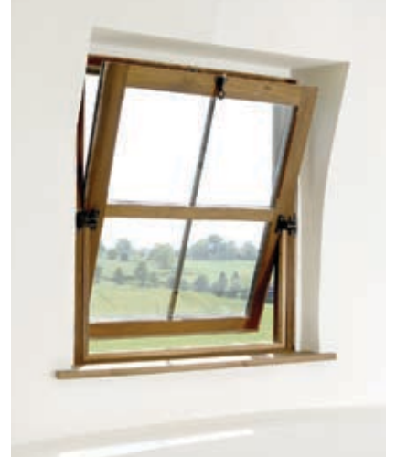
Oak centre pivot window, Staffordshire
