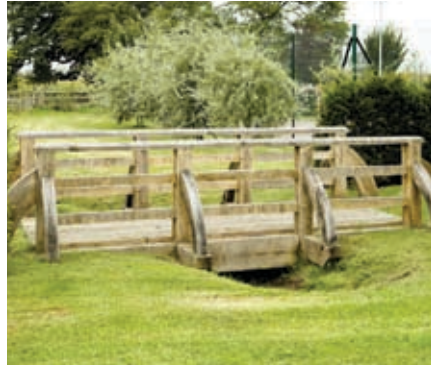
Oak bridge, Cheshire
